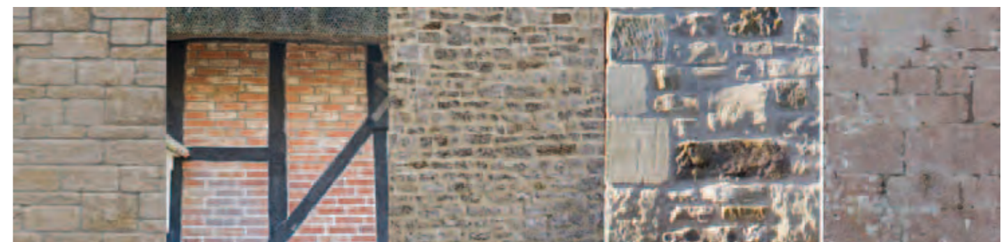
Below from left to right: reconstituted stone, brick nogging, lime pointing, reclaimed stone wall with squared quoins, Ashlar (hand cut stone). Opposite page above: View of the development adjacent to Barnmead. Opposite page below: mixed height roofs in Teffont Evias.
